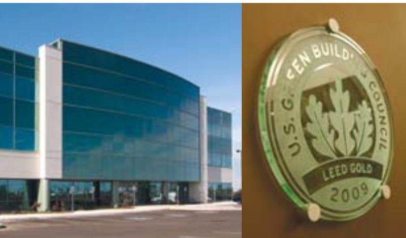
The Head Office of Penncorp and York Fire in Mississauga
